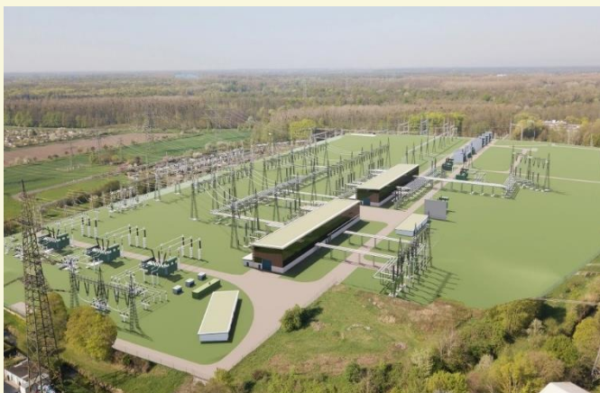
3D visualization of the new gas-insulated system – nitrogen/oxygen (N 2 /O 2 ) alternative gas mixture 'CleanAir' distributed by Siemens Energy
